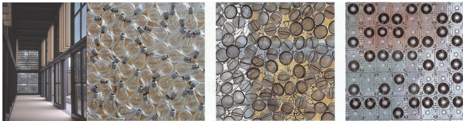
a) Von Gerkan’s Pavilion of Christ, internal view of the double envelope; b) the space between the glasses, filled with materials of various origins: from nature with coal, rush, bamboo, wood strips, feathers etc; from technology with toothed wheels, tea-strainers, hoses, lighters, lamps, one-way syringes. Depending on the filling the walls are more or less translucent, partially also transparent; consequently the light atmosphere is modified and varies dramatically along the cloister.
